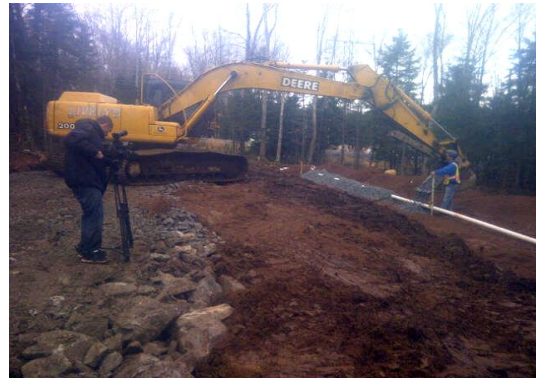
Figure 2: Installation of Gravel and Pipe Trench
